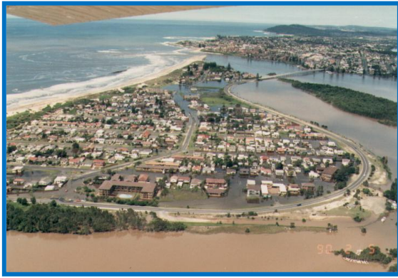
Entrance channel - February 1990 flood
