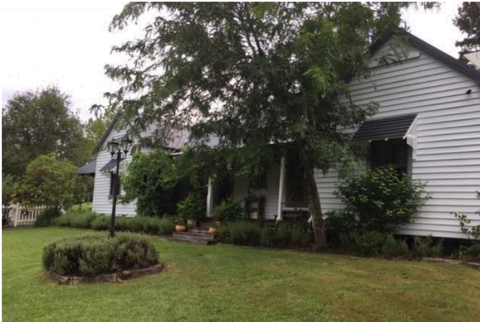
Photograph 8: Recent restoration works
