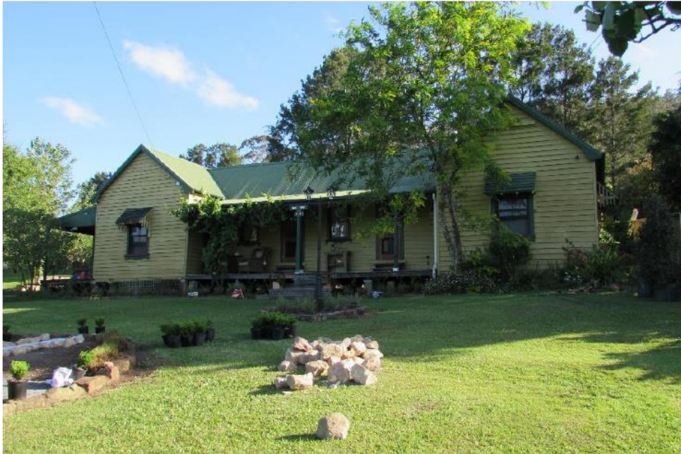
Photograph 3: Front of dwelling
