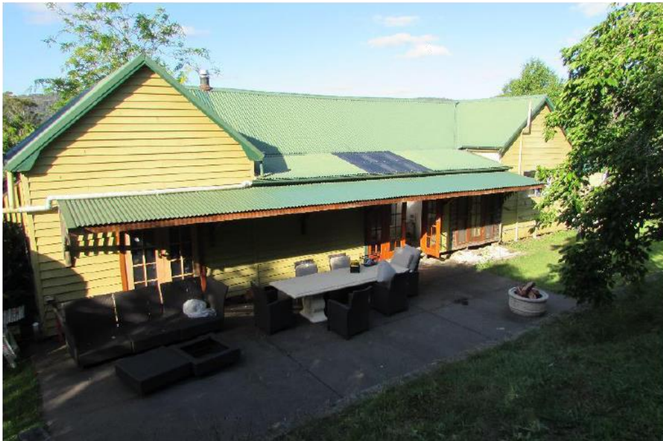
Photograph 4: Rear of house – the location of the approved extension
