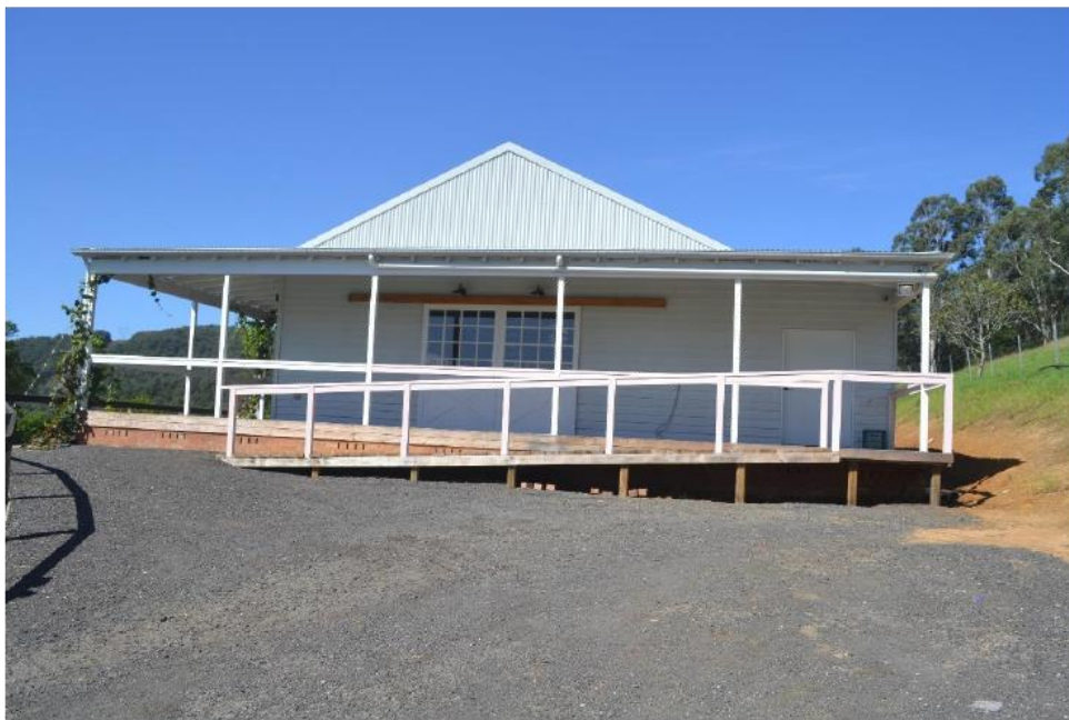
Photograph 9: Approved barn / shed
