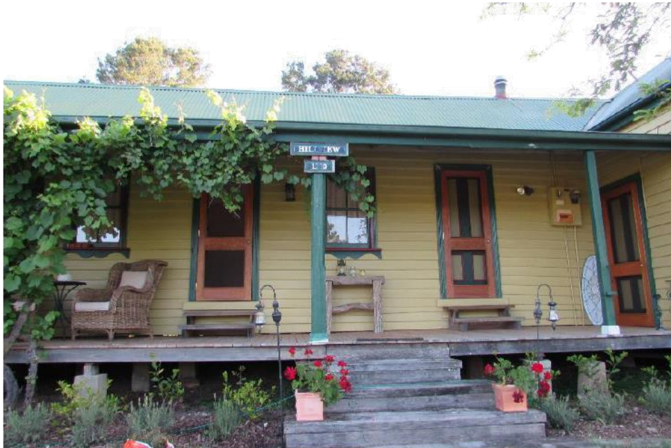
Photograph 5: Section of the house which is the original dwelling
