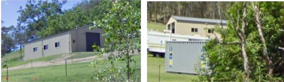
Figure 1 & 2 – Photos of shed at 1380 Yarramalong Road
