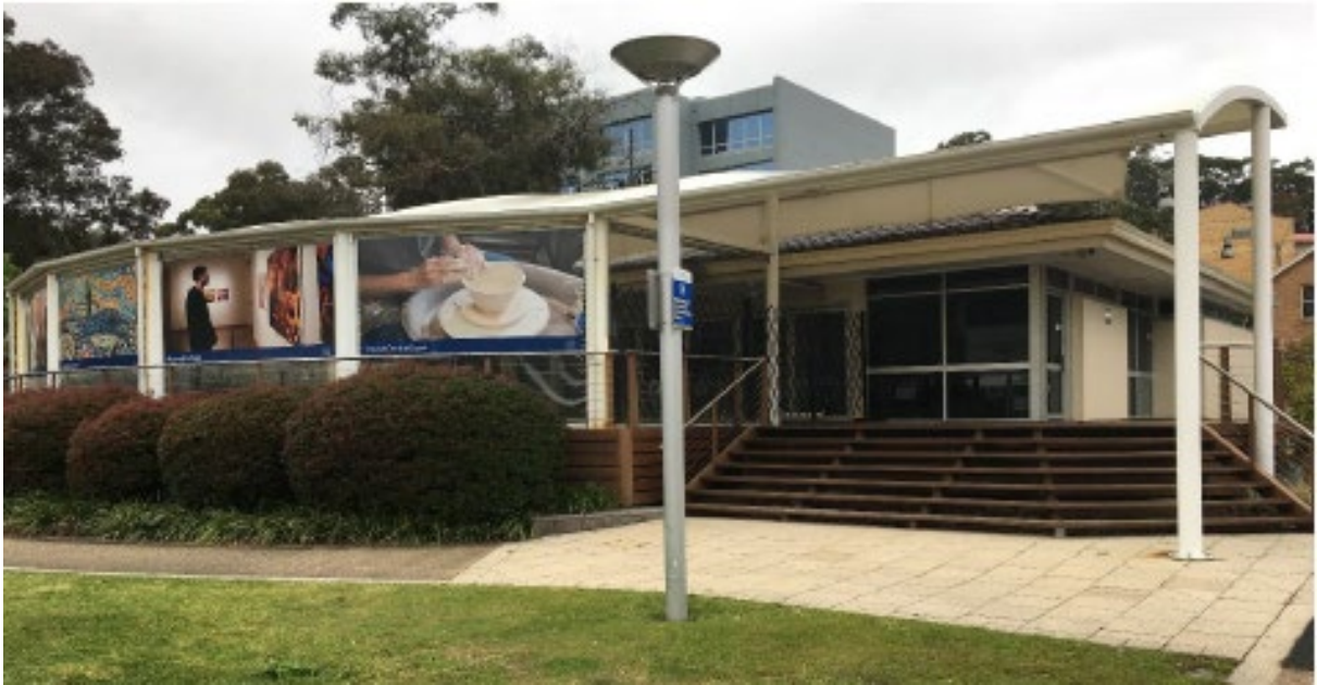
Figure 3- View of building from within Kibble Park
