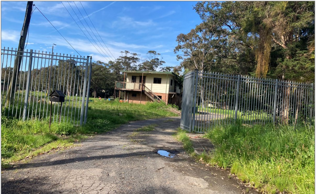
Figure 2 – Entrance to site via Bowtells Drive and southernmost dwelling
