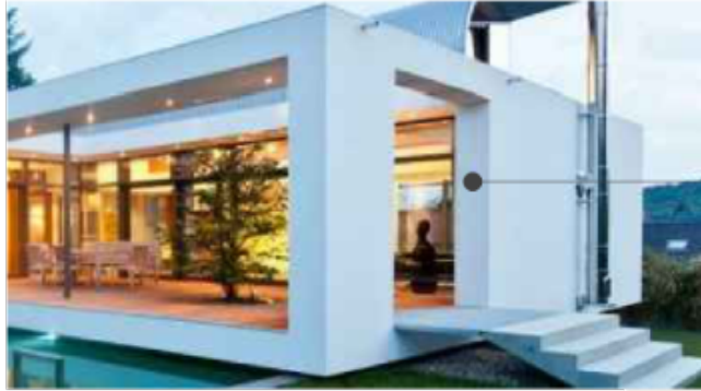
LIGHT STRUCTURE FRAME
