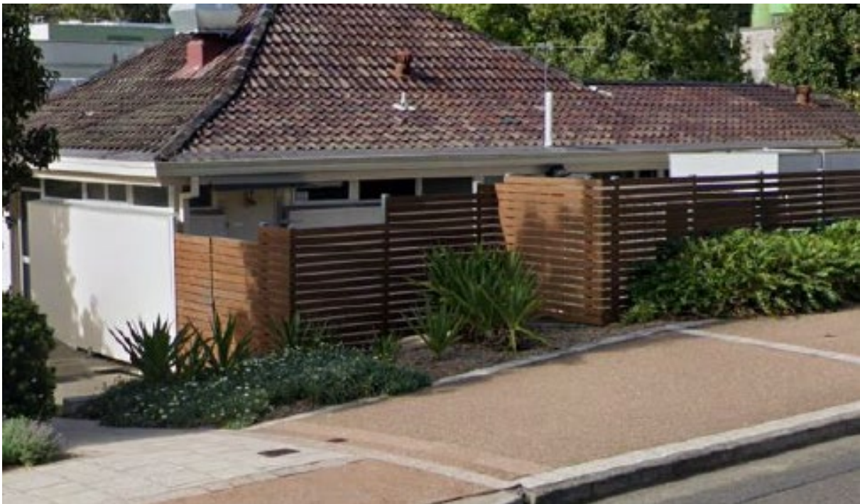
Figure 4- view of building from Donnison Street.
