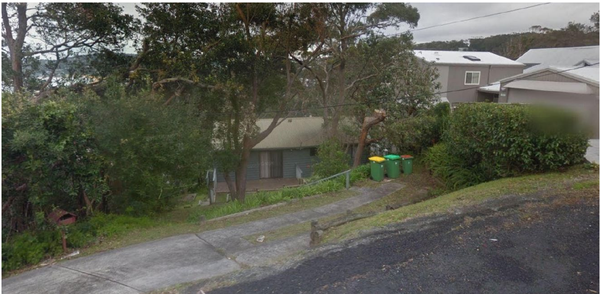
Figure3: Photo taken from road of existing weatherboard clad and metal roof dwelling proposed to be renovated.
