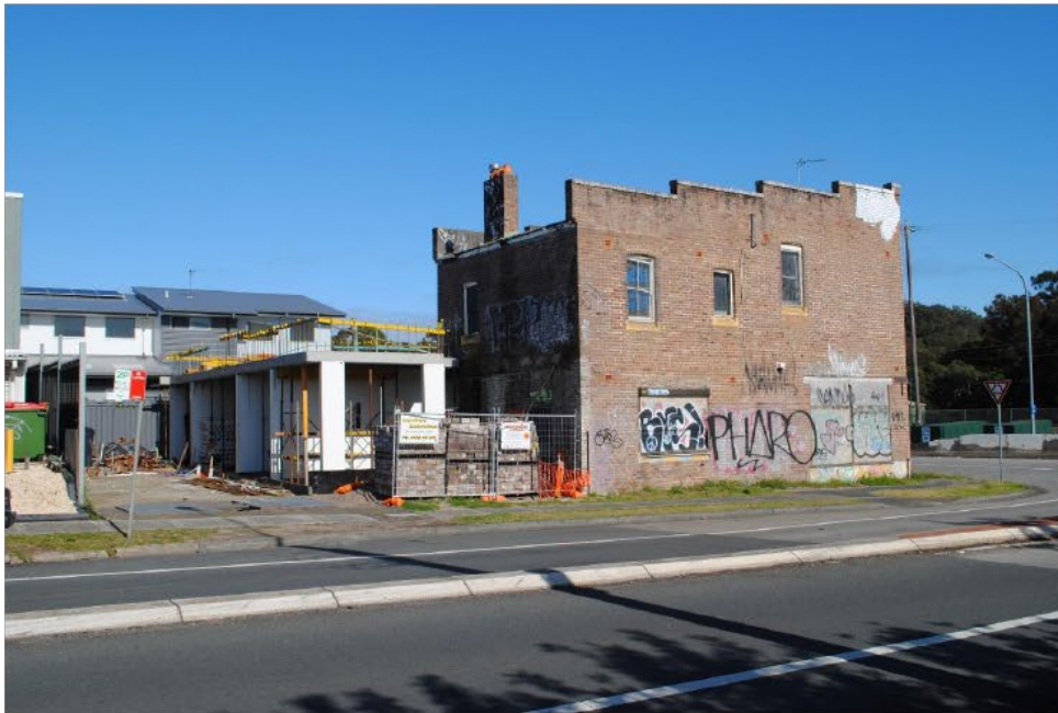
Figure 4 – Site viewed from Charlton Street
