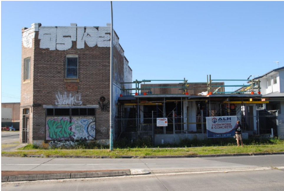
Figure 3 – Site viewed from Railway Street, with residential units under construction
