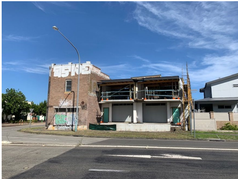
Figure 2 – Development under construction viewed from Railway Street
