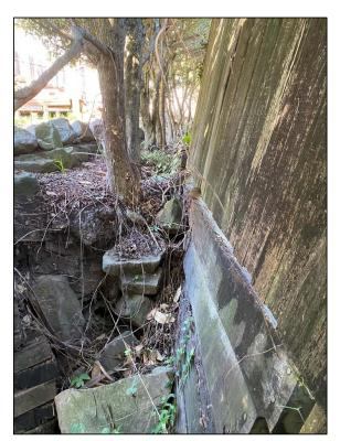
Photograph P3 – View of failed timber retaining wall along western boundary
