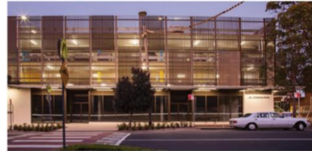
Padstow commuter car park, NSW (image: AW Edwards)
