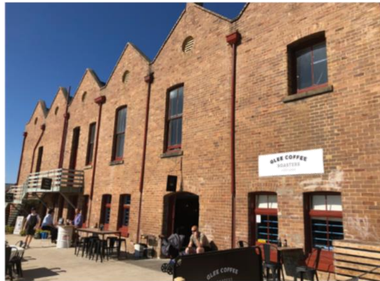
Chapman building, Wyong
