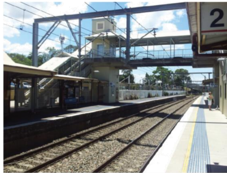
Wyong train station
