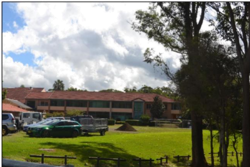
Photograph 4 – looking north at the site of the proposed building from the crossing of the culvert immediately to the south. The impact of the additional height of the building would be limited from this aspect due to the fact a public reserve is located immediately south of the culvert (see photograph 5 on next page).
