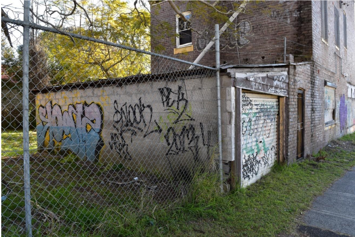
Figure 4 Photograph showing non-original single storey concrete block garage at the rear of the building
