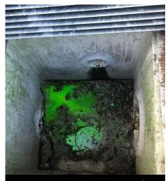
Dye tests - Ensuring unmapped connections are only stormwater
