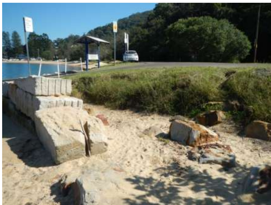
Figure 21 - Erosion observed behind the rock block seawall adjacent to the boat ramp
