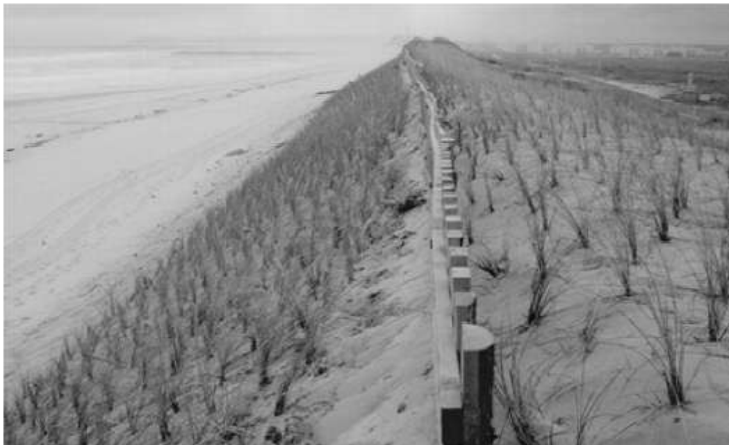
Figure 48 - Stabilisation of the dune by a dune fence and vegetation planting
