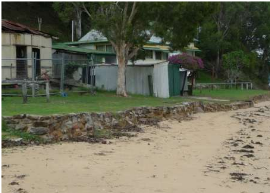
Figure 24: Mortared block seawall located in front of the houses in the Dark Corner
