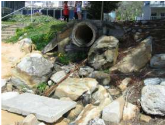
Figure 33: Ad-hoc protection placed in front of the stormwater outlet at 111 Avoca Drive (left) and scour in front of the stormwater outlet at 131 Avoca Drive (right).
