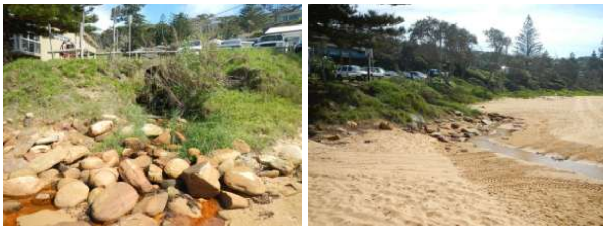
Figure 30: Rock boulders in front of the stormwater outlet near the MacMasters surf club (left) and scour channel from the outlet to the beach (right).
