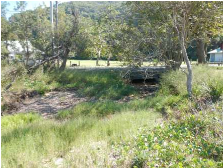
Figure 20 - Scour observed in front of stormwater outlet from Eve Williams Memorial Oval
