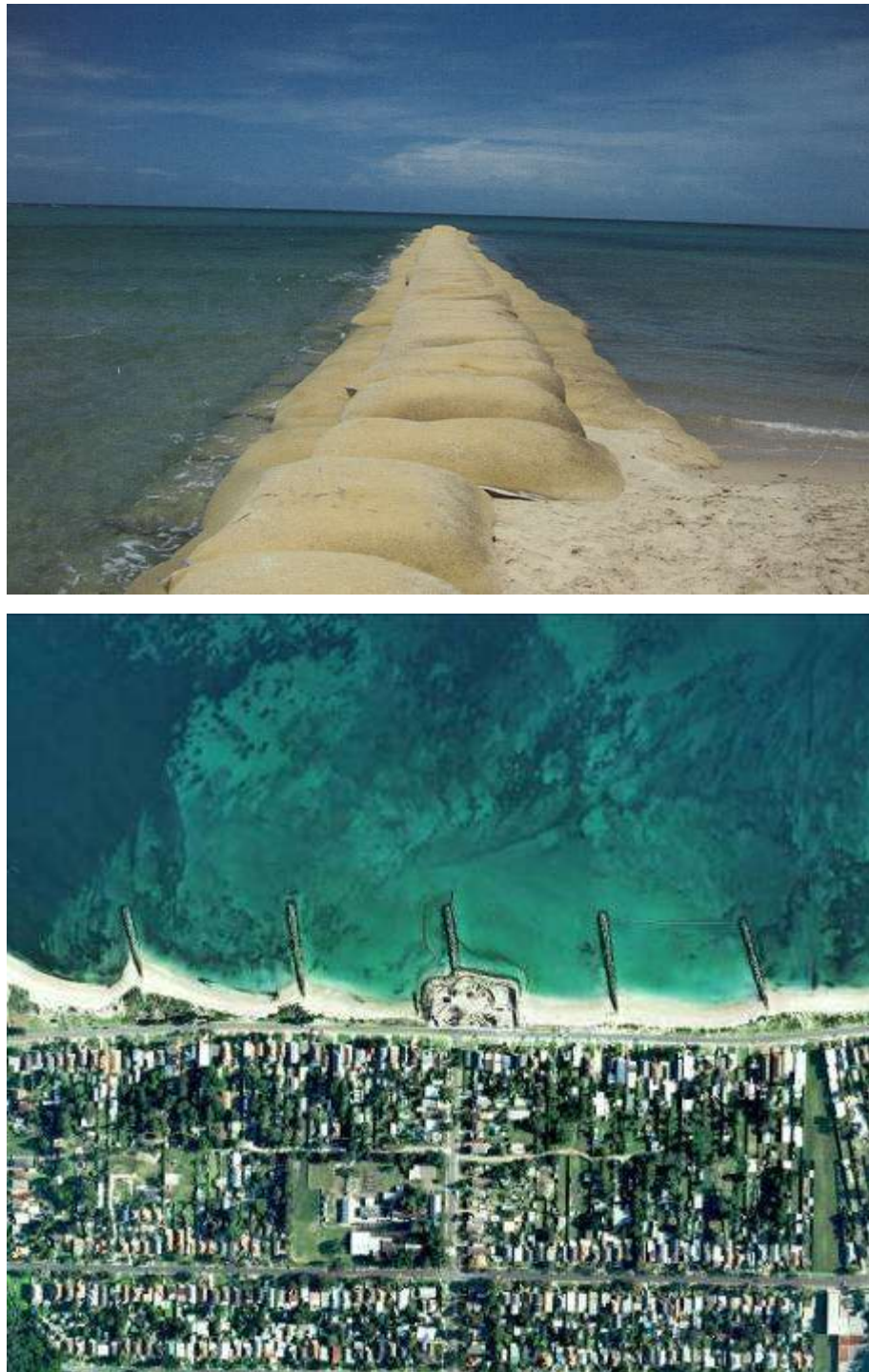
Figure 46 - Top - Example of a geotube groyne (Geofabrics Australasia Pty. Ltd.); Bottom – example of a groyne field at Botany Bay, NSW Australia showing the impact of the groynes on the planform of the beach.
