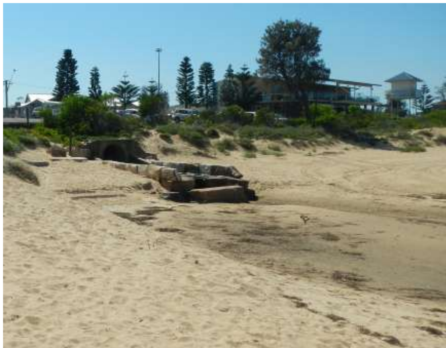
Figure 28: Sandstone block apron in front of stormwater outlet and scour in front of the apron.
