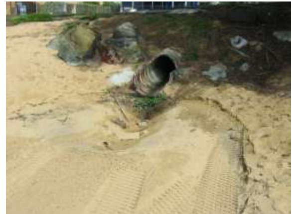
Figure 33: Ad-hoc protection placed in front of the stormwater outlet at 111 Avoca Drive (left) and scour in front of the stormwater outlet at 131 Avoca Drive (right).
