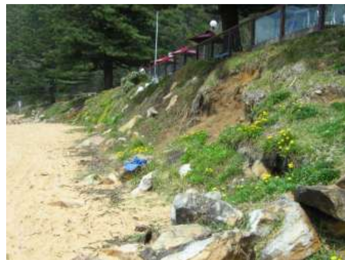
2. Ad-hoc erosion protection and embankment erosion along beachfront at MacMasters Beach Surf Club, 5 October 2010
