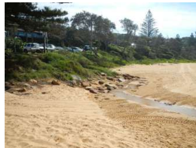
3. Scour at stormwater drain and weed growth over embankment, Marine Parade MacMasters Beach, 3 April 2014
