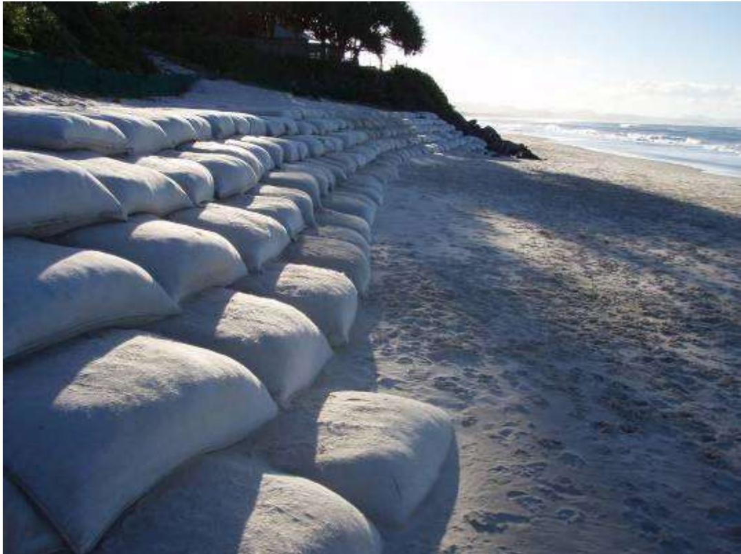
Figure 45 – Typical sand-filled geotextile container revetment at Byron Bay, NSW Australia
