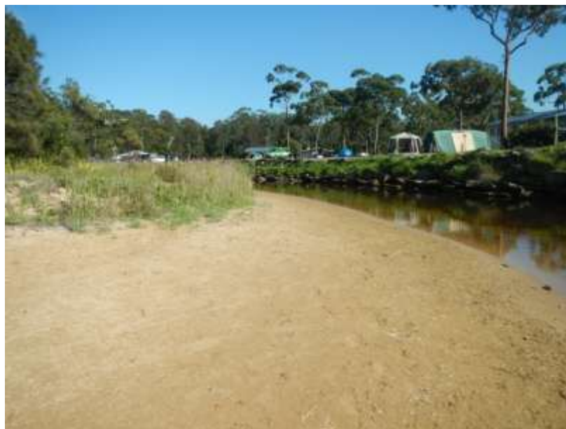
Figure 26: Rock boulder seawall on the northern side of Ettalong Creek and vegetated sand bank on the southern side of Ettalong Creek
