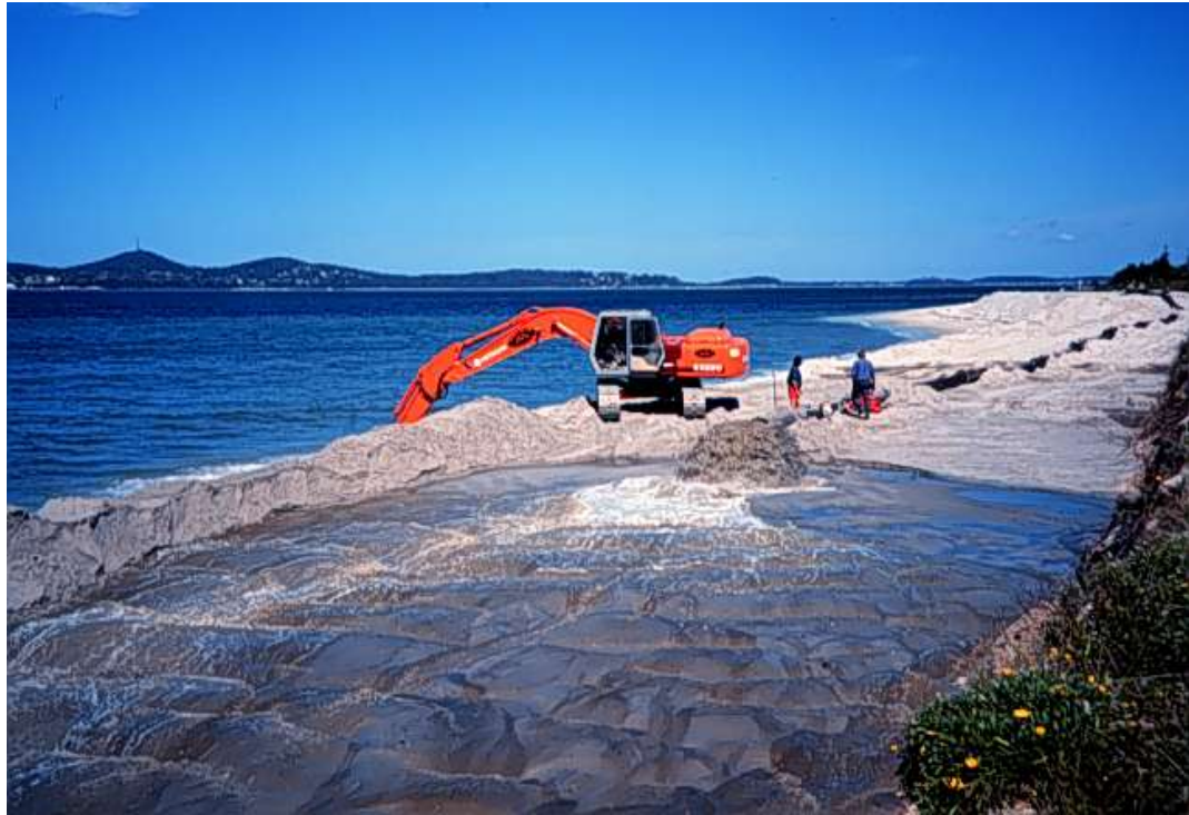
Figure 47 - Beach Nourishment construction, Jimmys Beach Port Stephens, NSW Australia
