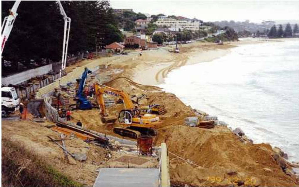
Figure 11: Construction of the sandstone block seawall at Terrigal Beach, December 1999 (photo courtesy Gosford City Council)
