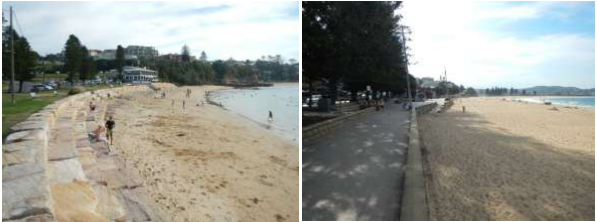
Figure 36: Stepped sandstone block seawall along the southern section of Terrigal Beach (left) and block seawall and promenade along the central section of Terrigal Beach (right)
