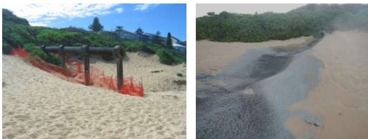
Figure 42: Piled stormwater outlet (left) replaced with a stormwater outlet within the dune system and a concrete apron in front of a stormwater outlet (right)
