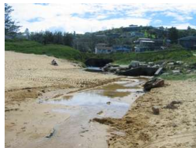
7. Scour at stormwater drain and creek entrance, near Copacabana surf club, 5 October 2010
