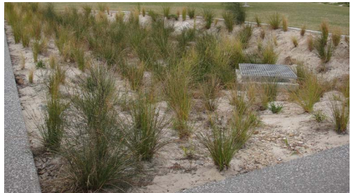
Example vegetated bio-filtration swale with raised pit
