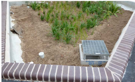
Example grassed swale with flush kerb
