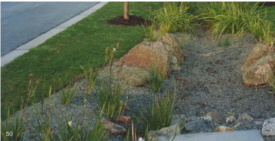
Example vegetated swale with flush kerb
