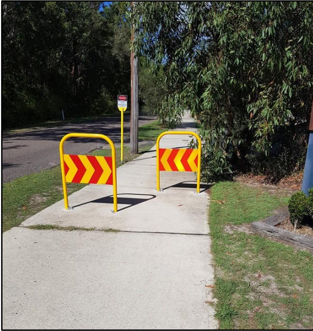
Figure 39: Incorrect shared path end treatment near driveway crossover
