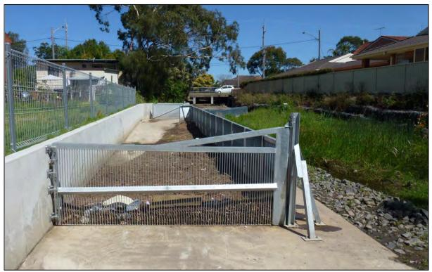
Plate 15 Example of Blockage Control Structure with "offline" debris accumulation bay
